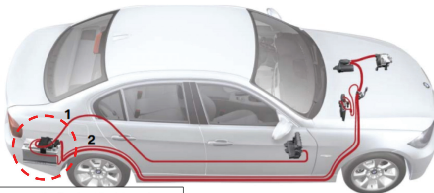
Power Distribution Block Location
